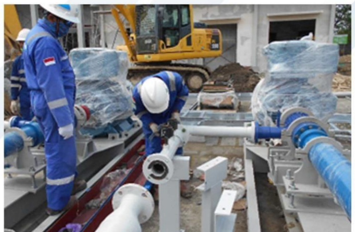
( Intalasi Piping & Pompa )
