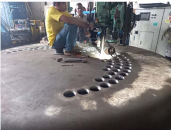
( Proses Drilling Tube Sheet Boiler )
