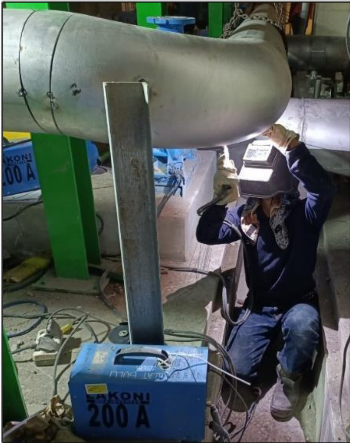
( Instalasi Piping & Welding )
