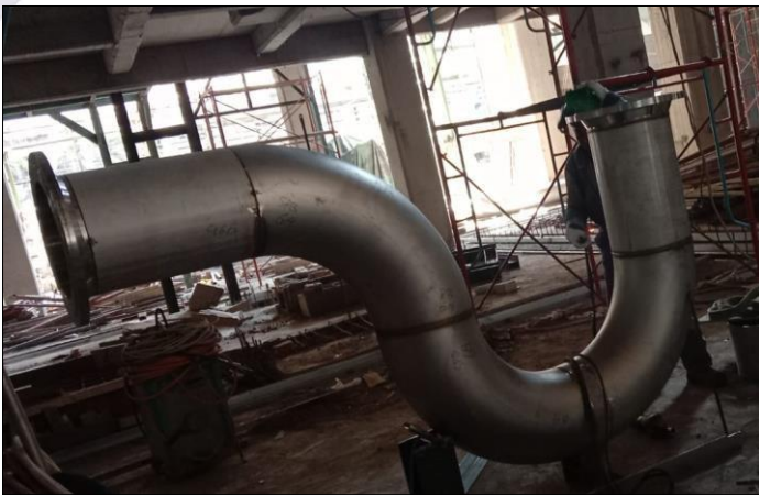
( Instalasi Piping Proses )
